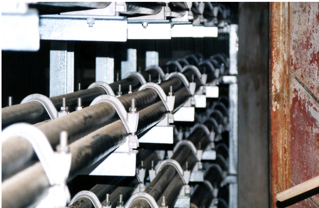
54 Series Fault Rated trefoil clamps carrying 33kV distribution cables in racked configuration
