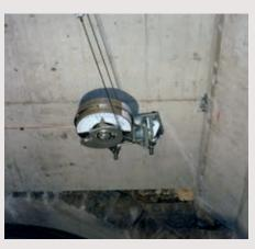
The spring tensioning system can be mounted directly to tunnel ceilings and rotated by up to 90°.
